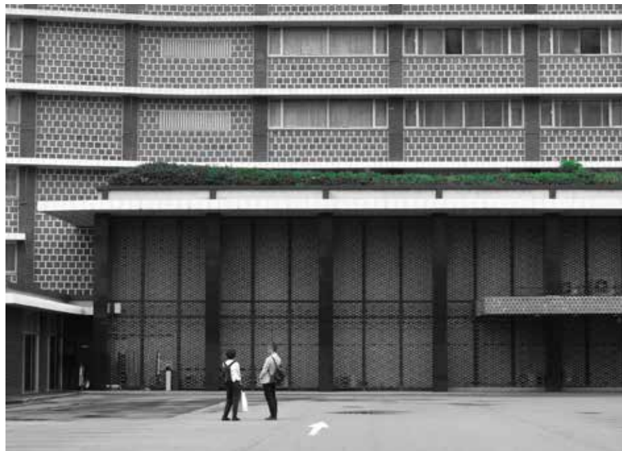
Hotel Okura, 1962: A modernist building most deserving of the label 'iconic', the Hotel Okura is sadly awaiting demolition, threatening the architectural history of the city.
