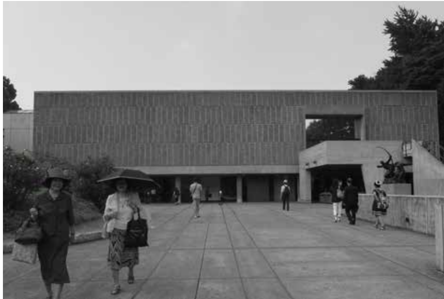
National Museum of Western Art, le Corbusier, 1959: Designed by Le Corbusier according to his prototype for a 'museum of unlimited growth', this building is the architect's only Far Eastern Work. This year, Unesco added it to a list of heritage buildings, together with 16 others designed by the great master.
