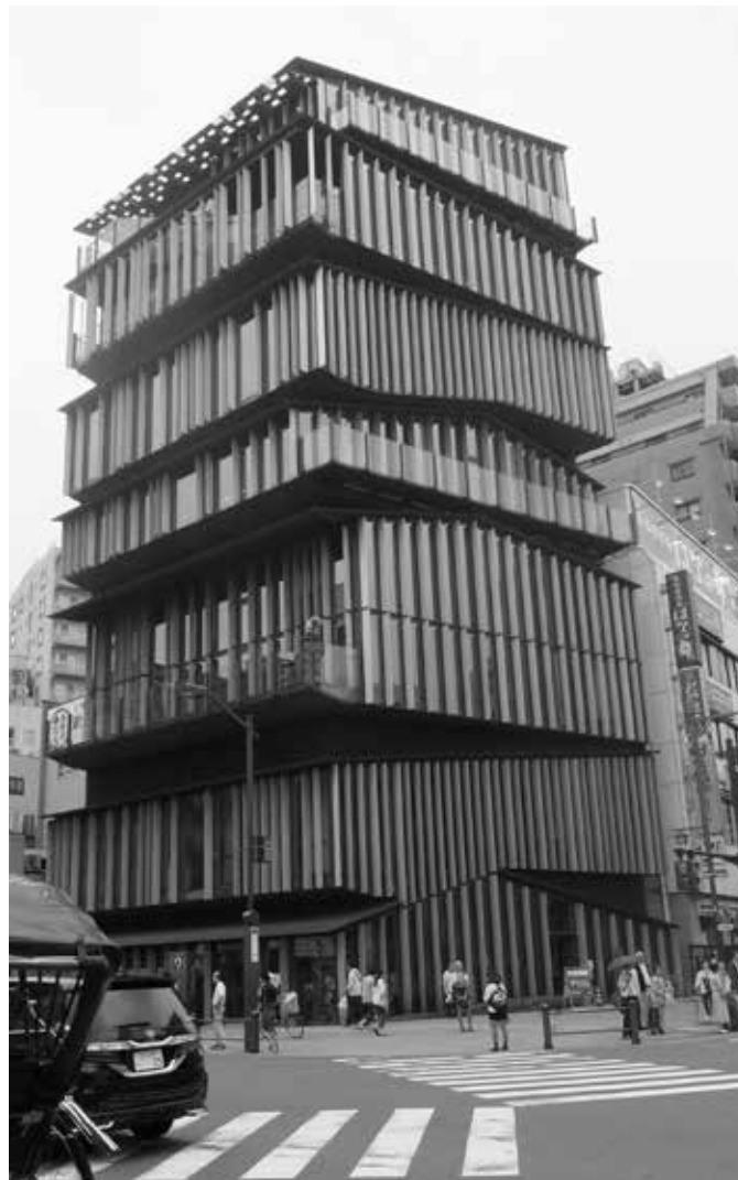
Kengo Kuma Culture and Tourism Centre, 2012: As an allusion to typical Japanese architecture, Kengo Kuma stacks up eight one-storey houses having a variety of sloping roofs.
